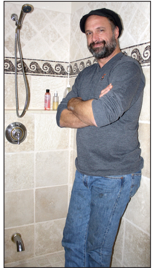
Bart Terwiel shows off a tiled shower project, including the toe tap for testing the water temperature.
