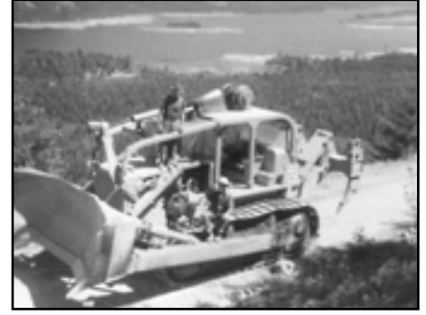
'Cat-skinning' near Cowichan.
